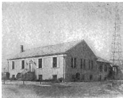
In this issue we are presenting some views of the WEAF transmitter equipment. This is the building which houses the main and emergency transmitters.
